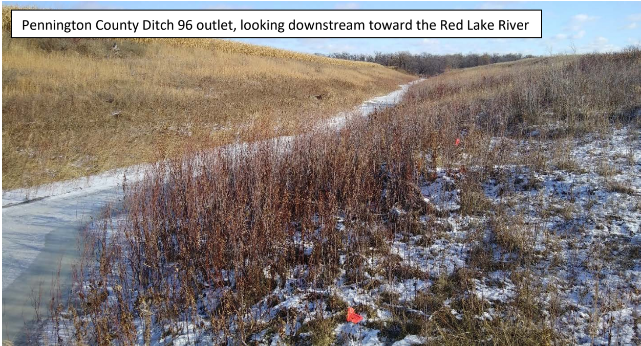
Stabilization of the CD 96 outlet will help preserve fish passage by preventing the downstream end of the Highway 32 culvert from becoming perched.
