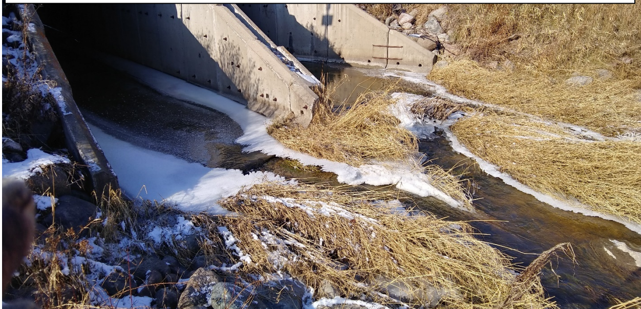
Stabilization of the CD 96 outlet will help preserve fish passage by preventing the downstream end of the Highway 32 culvert from becoming perched.
